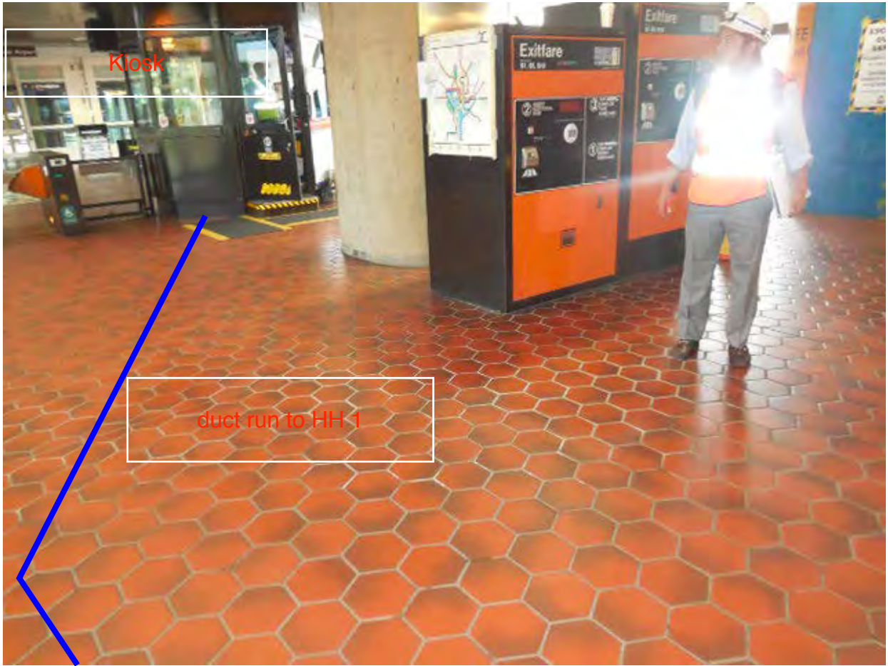
Photo #1 – C10 Reagan Airport North: Mezzanine Kiosk
